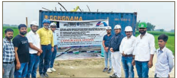
In Bihar, mainline hydrotest (HT-03 & 05) of cum. length 59.46 Km completed
