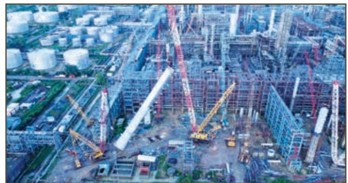
Erection of 1 st C3 Splitter Column(CC-3127) Bottom portion
