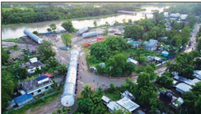
C3 Splitter Column (bottom portion) being transported from NRL Jetty to Site
