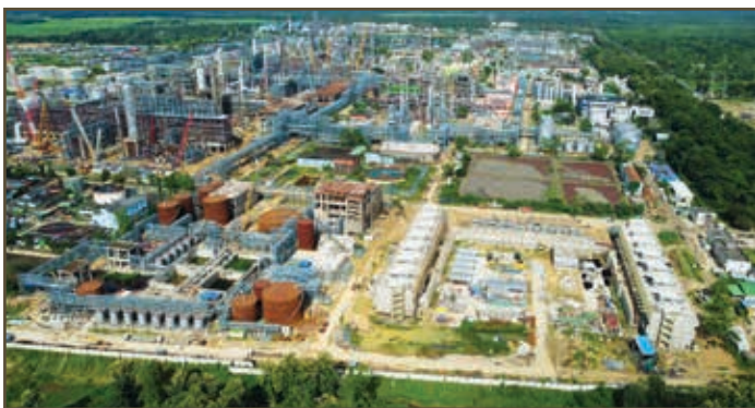
Overall view of NREP progress
