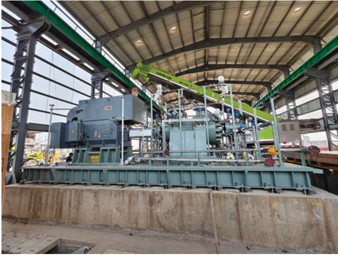
IPPS-01: 1 st Mainline Centrifugal pump erection on 25 th Feb'26
