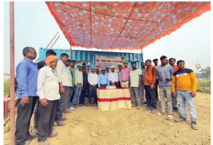
19.14 km mainline hydrotest from km 617(M-23) to km 636(M13)) Completed on 11 th Mar'26 in Part-C (Jharkhand)
