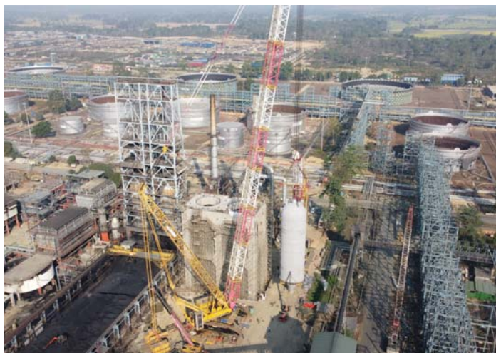
Coke Drum Erection
