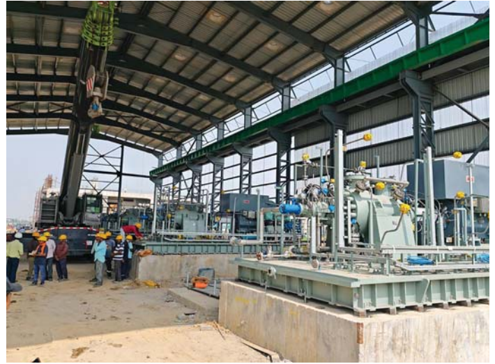
IPPS-01: Erection of all mainline pump
