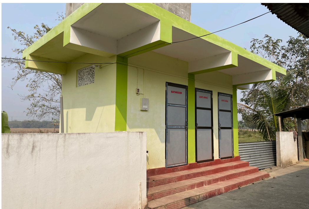
Fig. 29 - Toilets constructed under Project Parichannata
