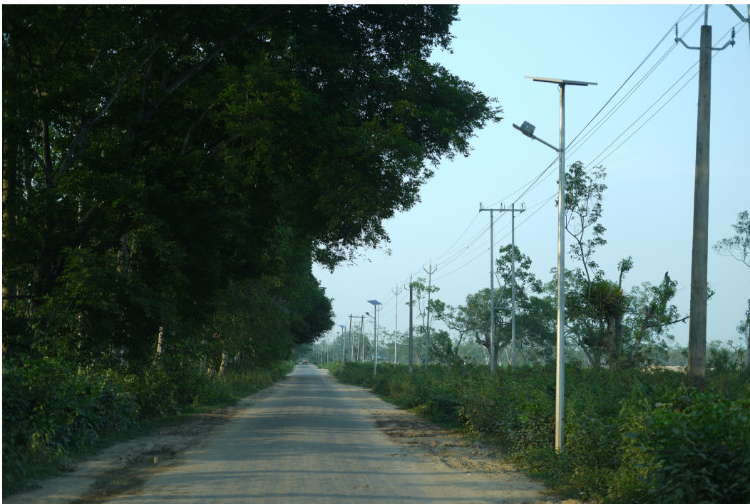
Fig. 26 - LED solar street lights
