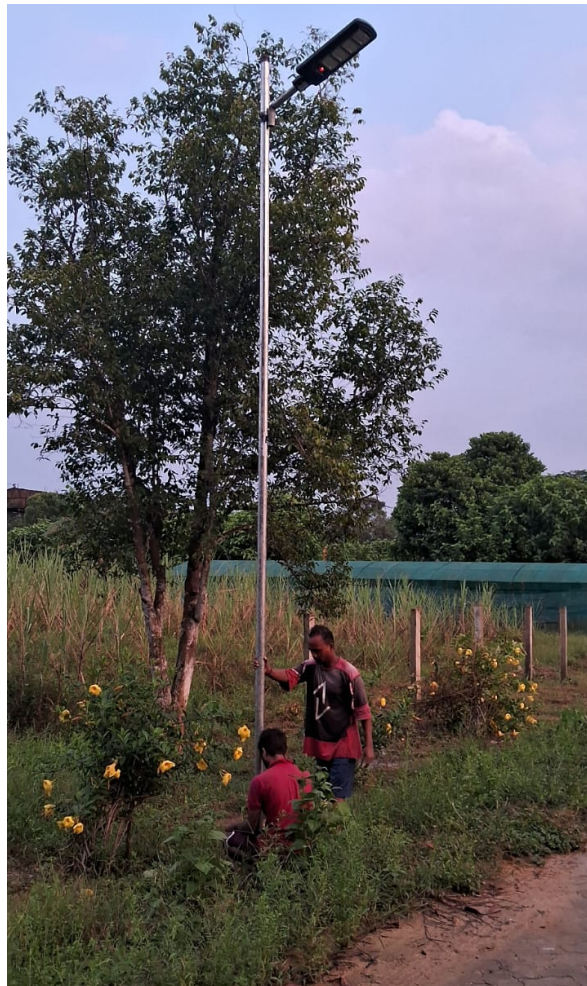
Fig. 27 - Installation of solar street lights
