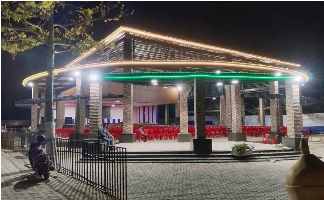
Fig. 31 - Open air auditorium constructed at Sarupathar
