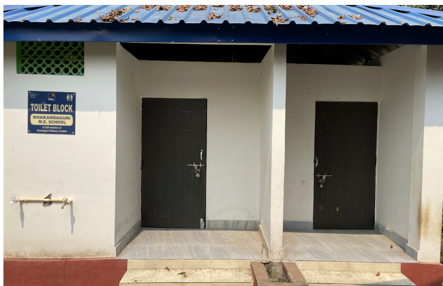
Fig. 28 - Toilets constructed at Khakandaguri M.E. School
