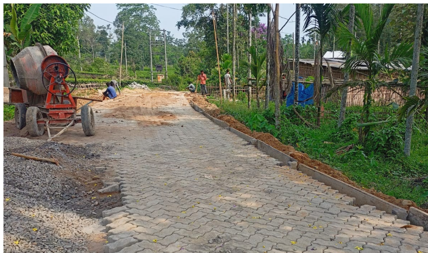
Fig. 30 - Rural roads construction at Rongbong
