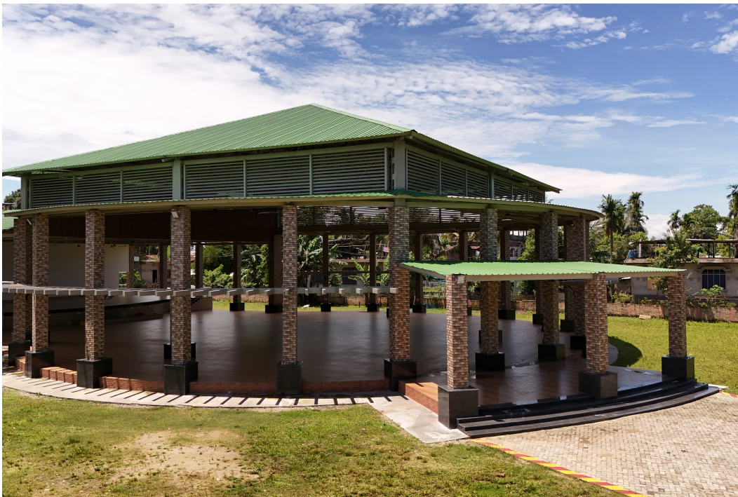
Fig. 33 Auditorium constructed at Bokakhat Town
