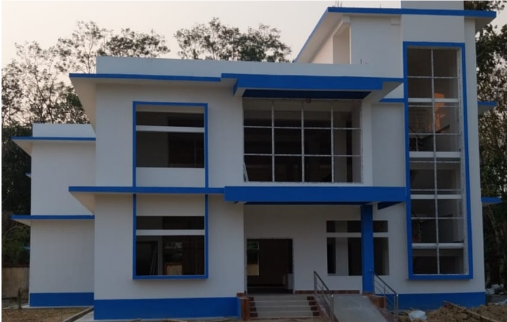
Fig. 21 - Library cum Wellness Centre under construction at Sarupathar College
