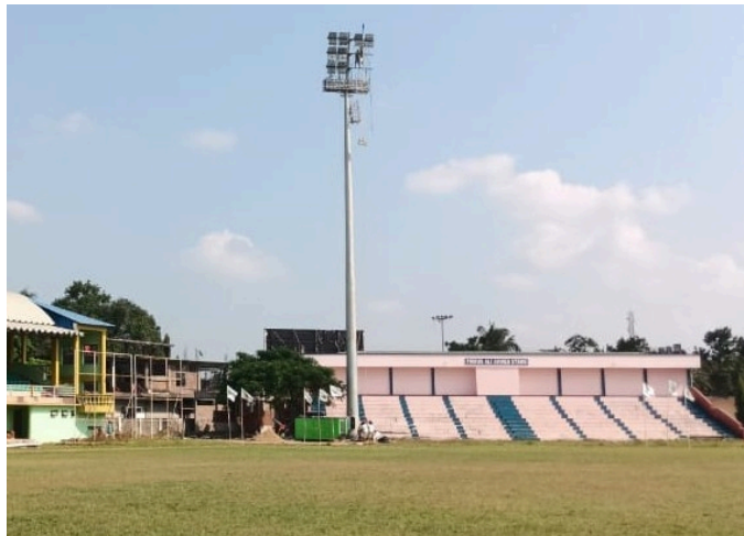
Fig. 2 - Flood light at GDSA Stadium, Golaghat
