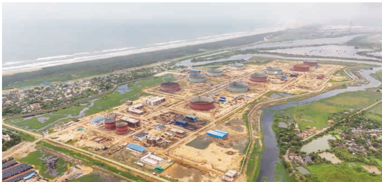
Crude Oil Import Terminal, Paradip
