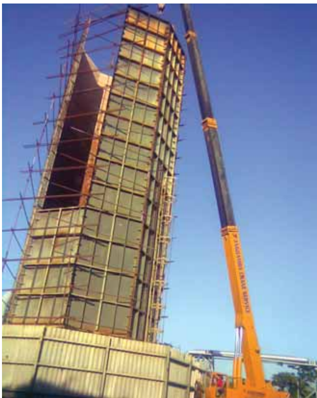
Ground flare panel refractory renewal job in progress during RTA 2008
