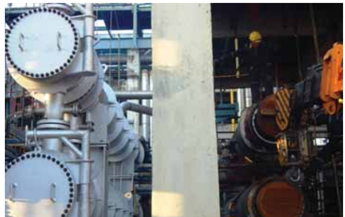
Installation of Pumps & Exchanger
