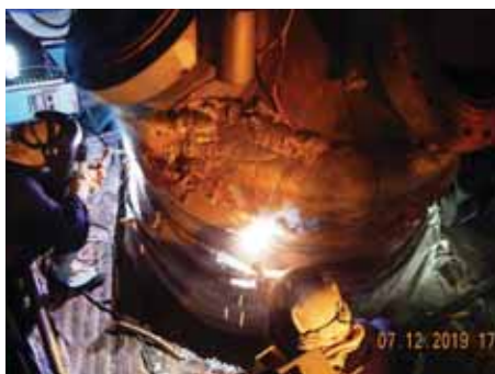
Packinox Exchanger Dish-end Welding Job
