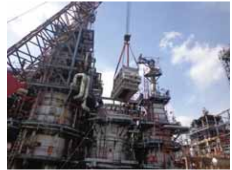
Removal of Old Heater (15-FF-03)
