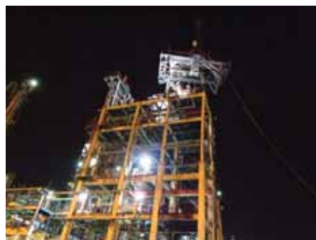
Dismantling of AFC structure
