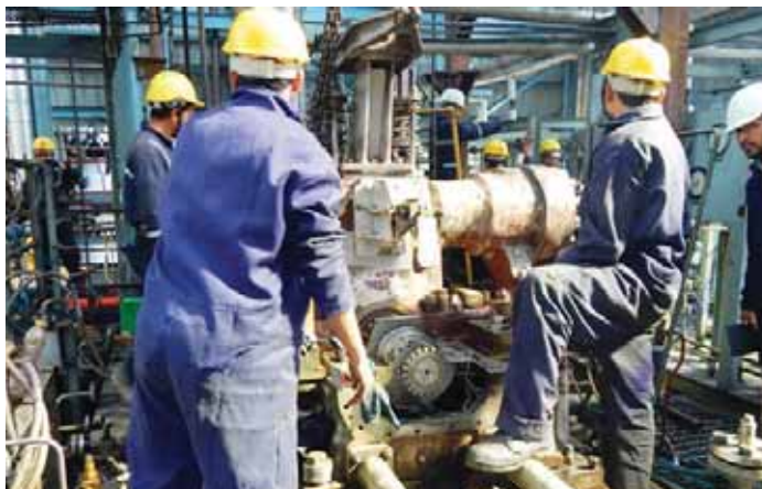
Installation of Pumps & Exchanger
