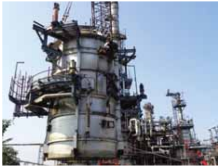
Removal of Old Heater (15-FF-03)
