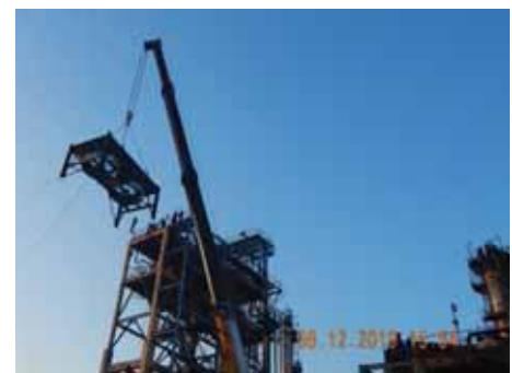
Erection of Air Fin Cooler
