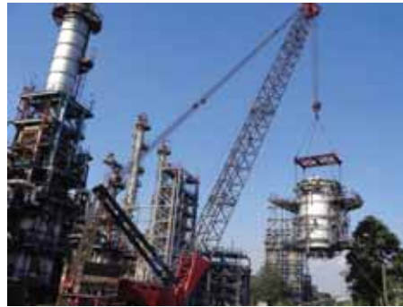
Erection of Heater Radiant Section (15-FF-04)
