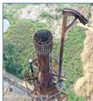
Inspection of elevated flare by drone
