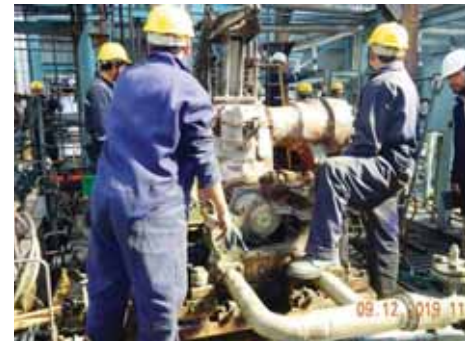
Recycle Gas Compressor Revamp Job
