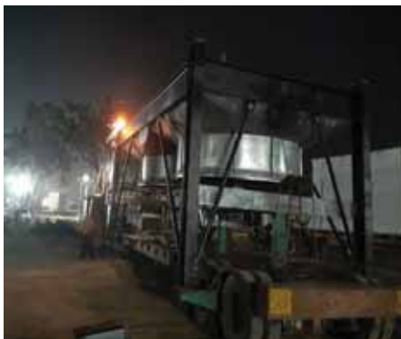
Modification of modular structure for Air Fin Cooler in Aurangabad
