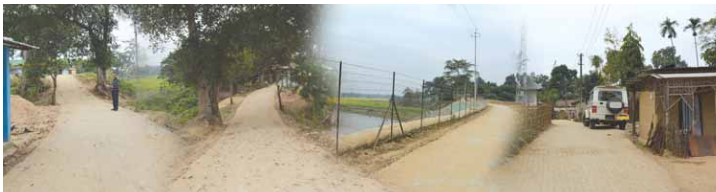
Numaligarh Block Gaon earned a face lift with all road renovations completed during the quarter
