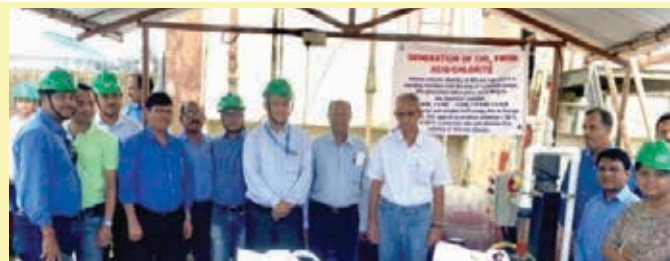
A chemical treatment facility for part reuse of treated effluent water in fire water network installed and commissioned on 26th September 2019, making BCPL a zero discharge plant.
