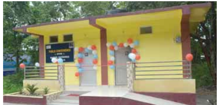
Public Toilet facility inaugurated at Bagori, Kaziranga National Park (13.07.18)
