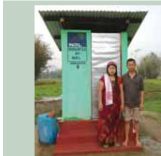
Toilets constructed in Direct Beneficiary Transfer (DBT) mode for making villages open defecation free (ODF)
