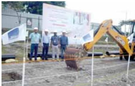
Groundbreaking of India Bangladesh Friendship Pipeline at Siliguri Marketing Terminal, NRL
