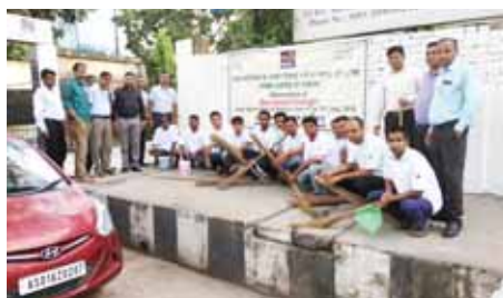
White washing of roadside boundary wall in Guwahati ( 14.07.18)
