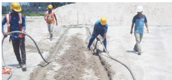
Anode laying for CP system along with PVC liner and Leak detection pipes laying completed in Tank No. 0703
