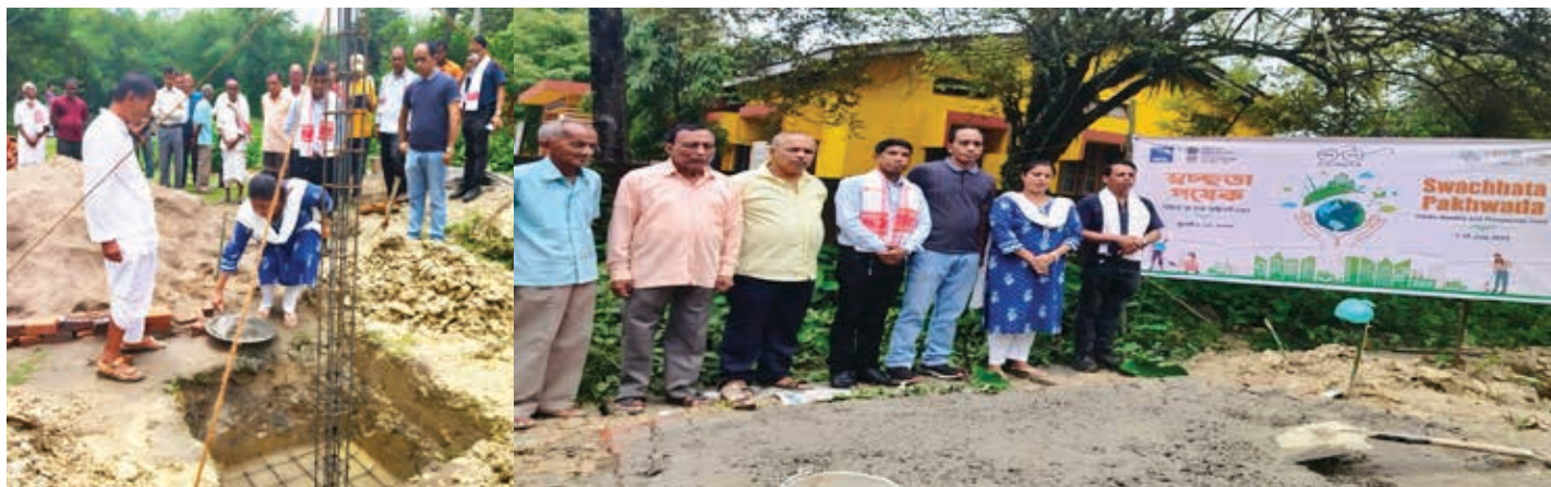
Foundation-laying of Public Toilet at Kuralguri Primary Health Centre (PHC), Dergaon in Golaghat district on 2 nd July, 2023 in presence of NRL representatives, Village Head, Medical officer and staff of the PHC
