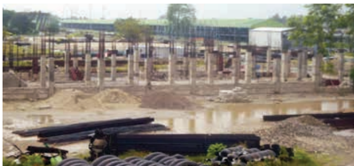
All the RCC columns for the 33 kVA substation building up to first-floor height have been accomplished during this quarter
