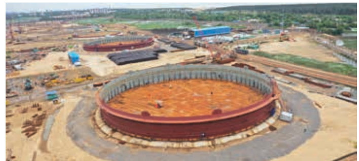
Mechanical works being carried out in full swing at Tank 409 & 410 (COIT Paradip) during September, 2023
