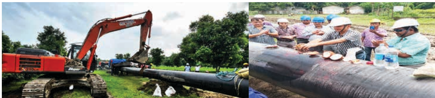
Mainline Pipe dumping & stringing works started at site (Ch. 866 Km) Laldas, Darjeeling on 27 th July, 2023
