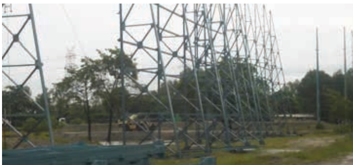
Erection of 45 barricading structure has been completed in the New Tank Farm area
