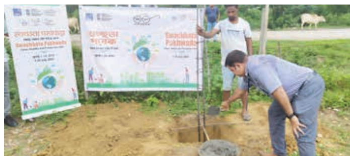
Foundation laying ceremony for toilet block at Bogidhola Muga VGR on 13 th July, 2023
