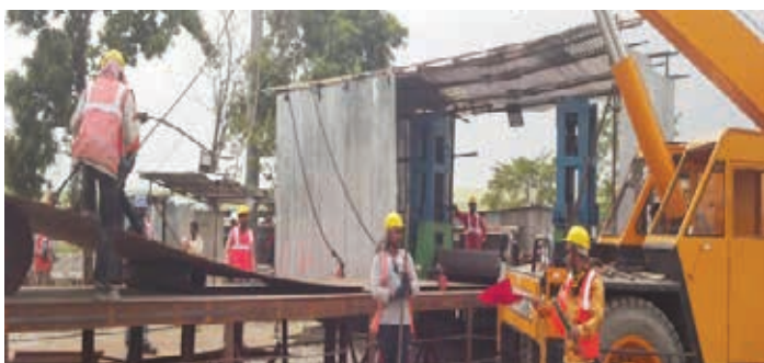
Fabrication of Tank Bottom, Annular, and Shell plates for Tank No. 0703 (MS), 1601 (SLOP) & 1602 (SLOP) completed
