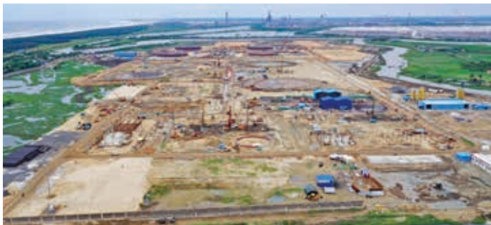
Bird eye view for Crude Oil Import Terminal (COIT) as on September, 2023
