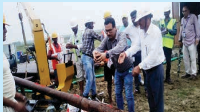
Pilot boring for 1 st HDD of PNCPL by CIPL at River Nunia, Odisha on 1 st July, 2022
