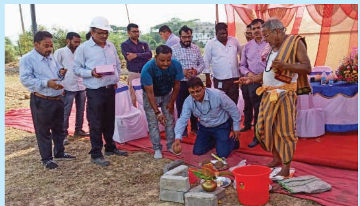
Director (Finance) Mr. Indranil Mittra performing Bhumi Pujan for setting up of civil construction of first SV station (SV-11) of PNCPL at Hidigaon, Balasore, Odisha
