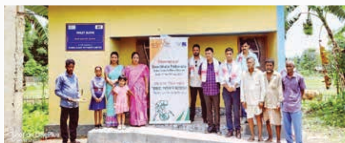
Toilet blocks inaugurated in two schools, namely Madhupur LP School, and Garamur Bortika LP School under Golaghat district of Assam in the presence of NRL Officials, School management committee members and teaching staff on 6 th July, 2022
