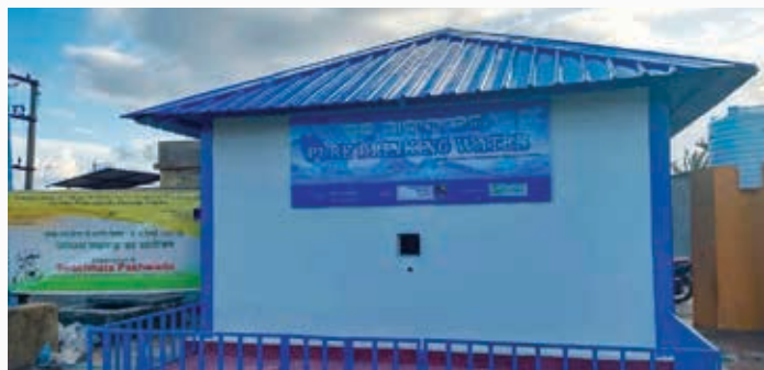
2 RO Drinking Water Plants (1000 LPH Capacity) installed under Sandhakuda Municipal area at Paradip, Odisha, on 12 th July, 2022, which will benefit almost 8,000 people
