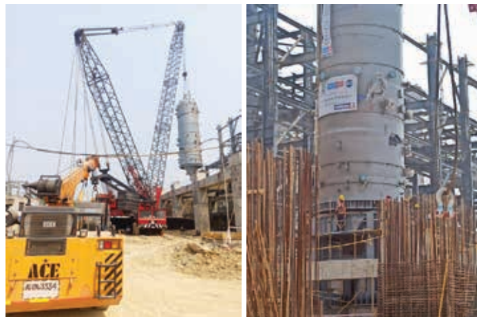
Erection of the 1 st Digester package at Numaligarh on 18-03-22
