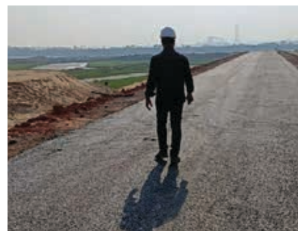
First Bitumen road at Crude Oil Import Terminal (COIT) completed on 21 st February 2023.
