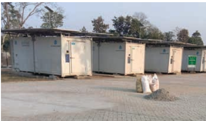
Development of Solar cold Storage site at Panbari, Bokakhat
