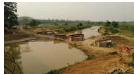
Construction of additional bridge in progress on Kaliyani river
