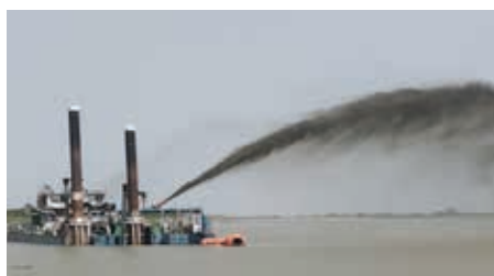
Dredging job is in progress in Dhansiri River
