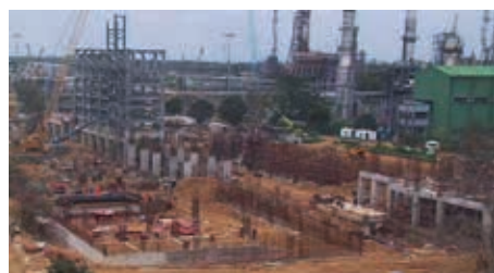
Civil & structural Job in DHT unit
