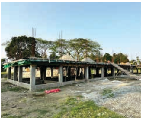
Ongoing construction work at Dusutimukh State Dispensary, Golaghat
