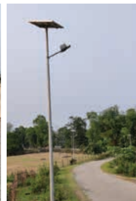
Installation of 400 Solar street lights in Golaghat and Dibrugarh District during March'2023.
