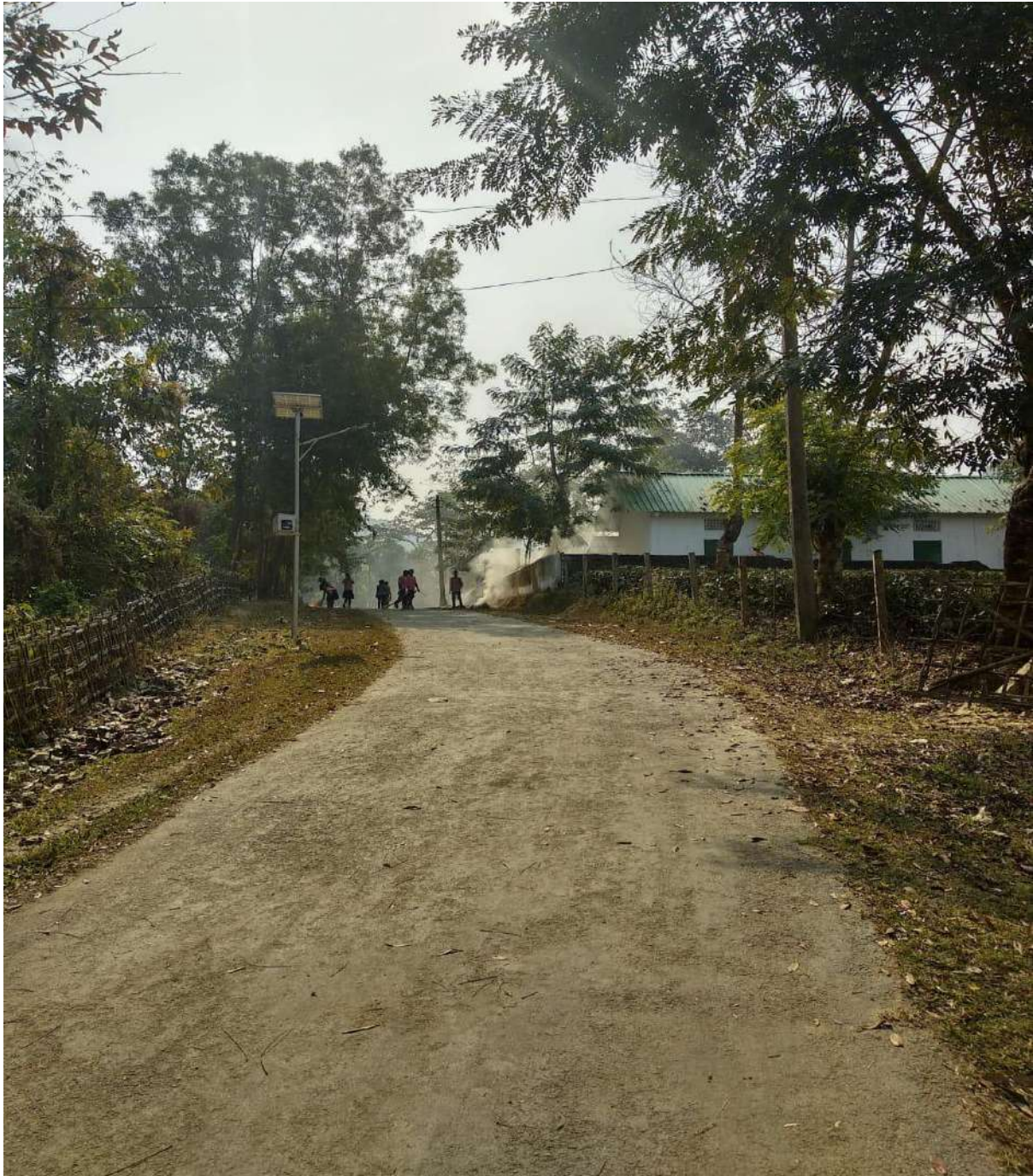
Image 19 Road constructed by NRL
