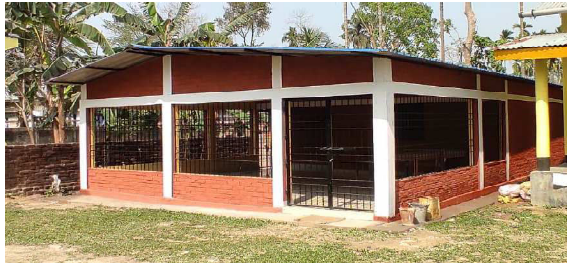
Photograph of Sl. No. 4 (a): Construction/ Renovation of Anganbari Kendra
