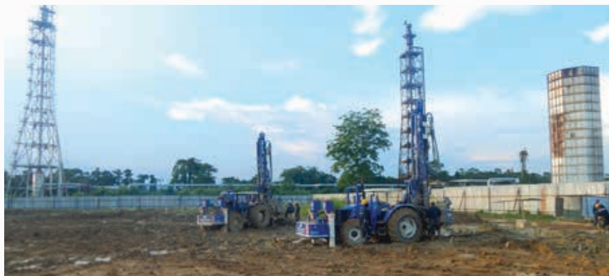
Site development work for ongoing Refinery Expansion Project
