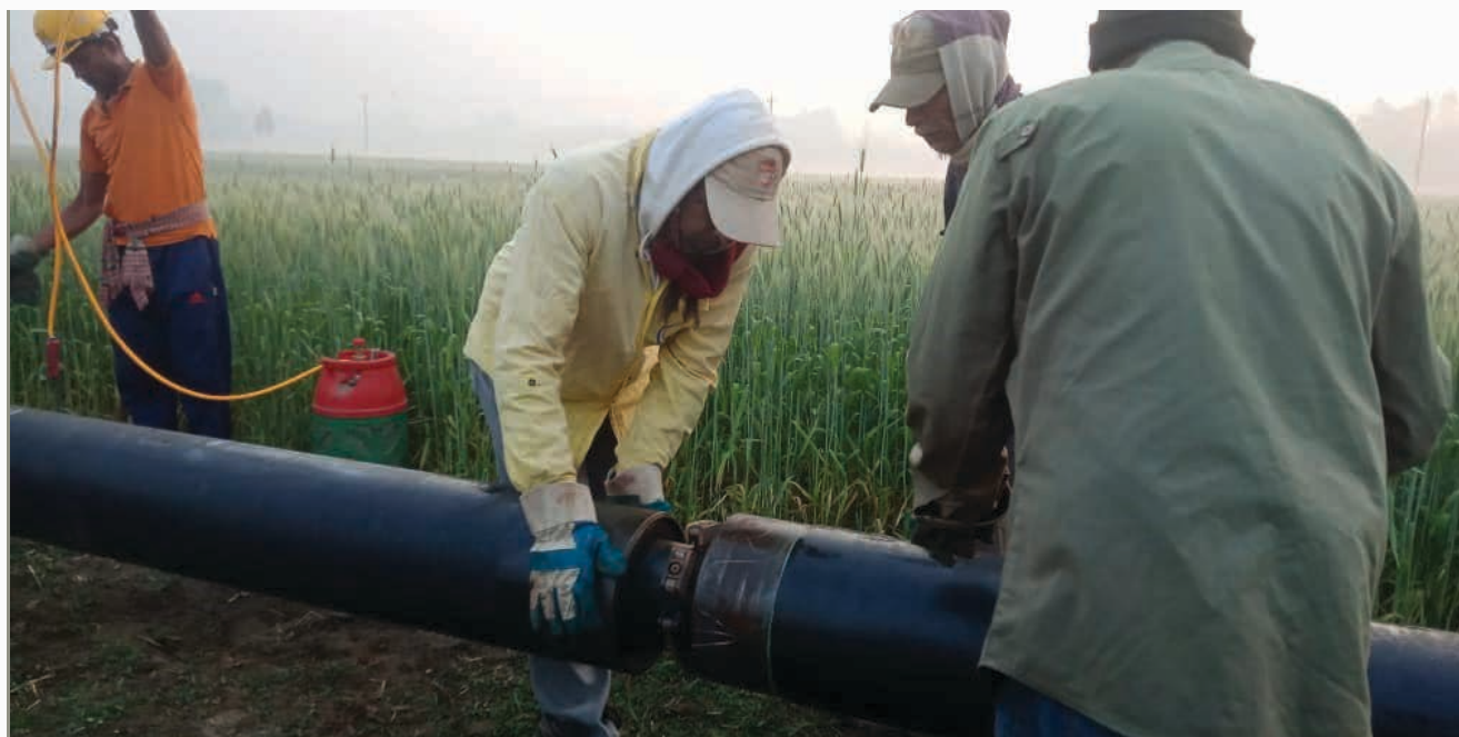
India Bangladesh Friendship Pipeline (IBFPL) work in progress
