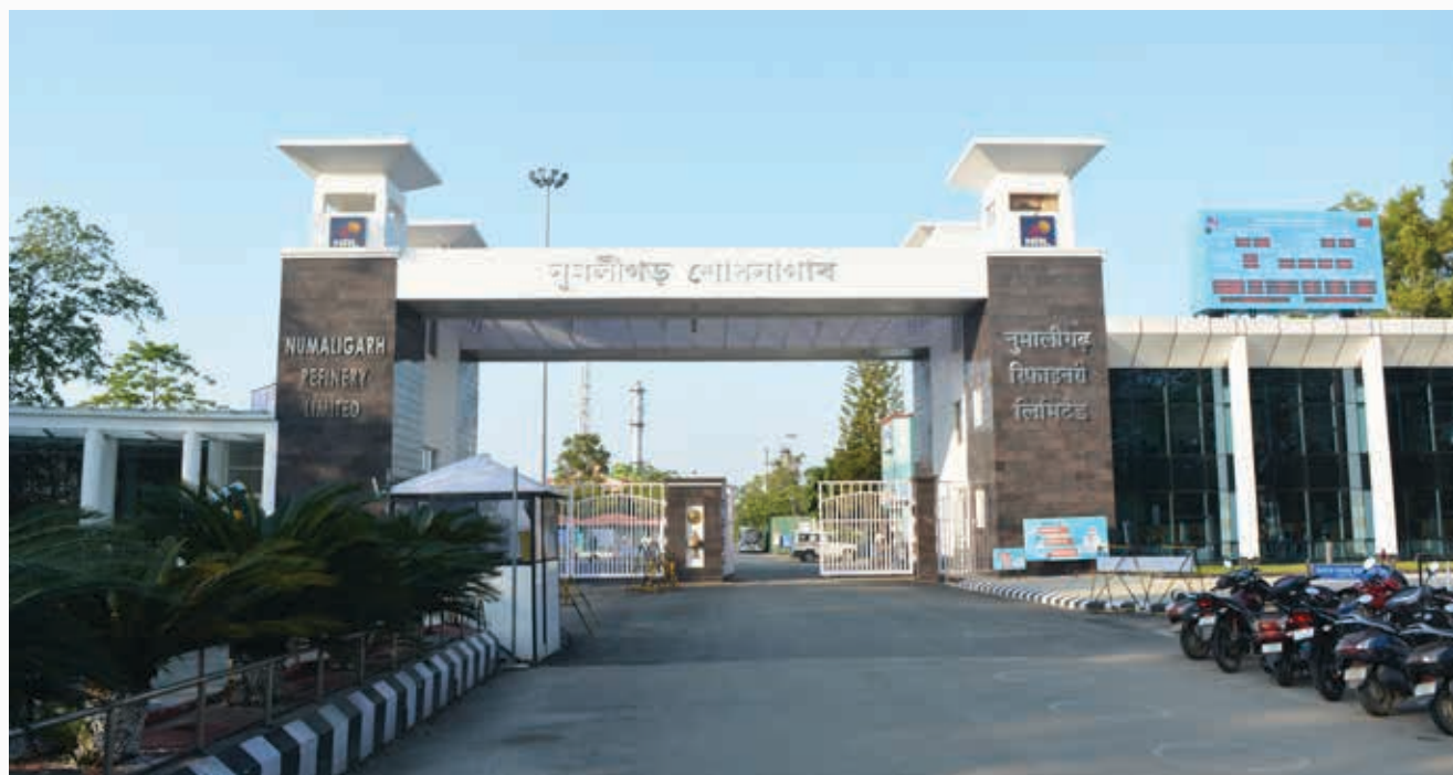
Newly inaugurated Refinery Main Gate
