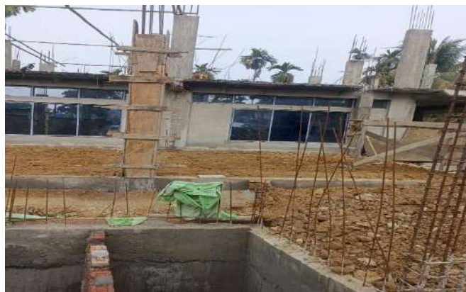
Ongoing Construction work Library Cum Learning Centre at Letekuchapori
