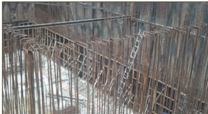
Foundation work in progress for Ethanol Sump UG vessel
