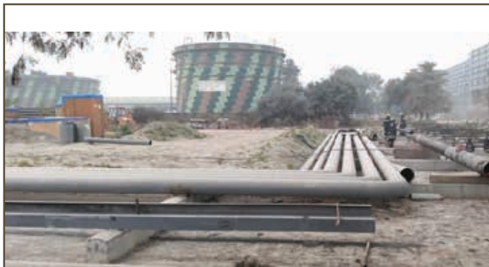
Erection of process pipes at SMT as part of Augmentation Work
