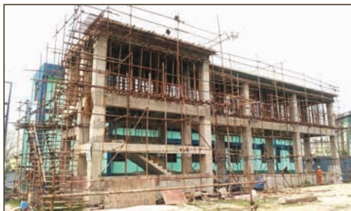
UPS cum Battery Room construction
