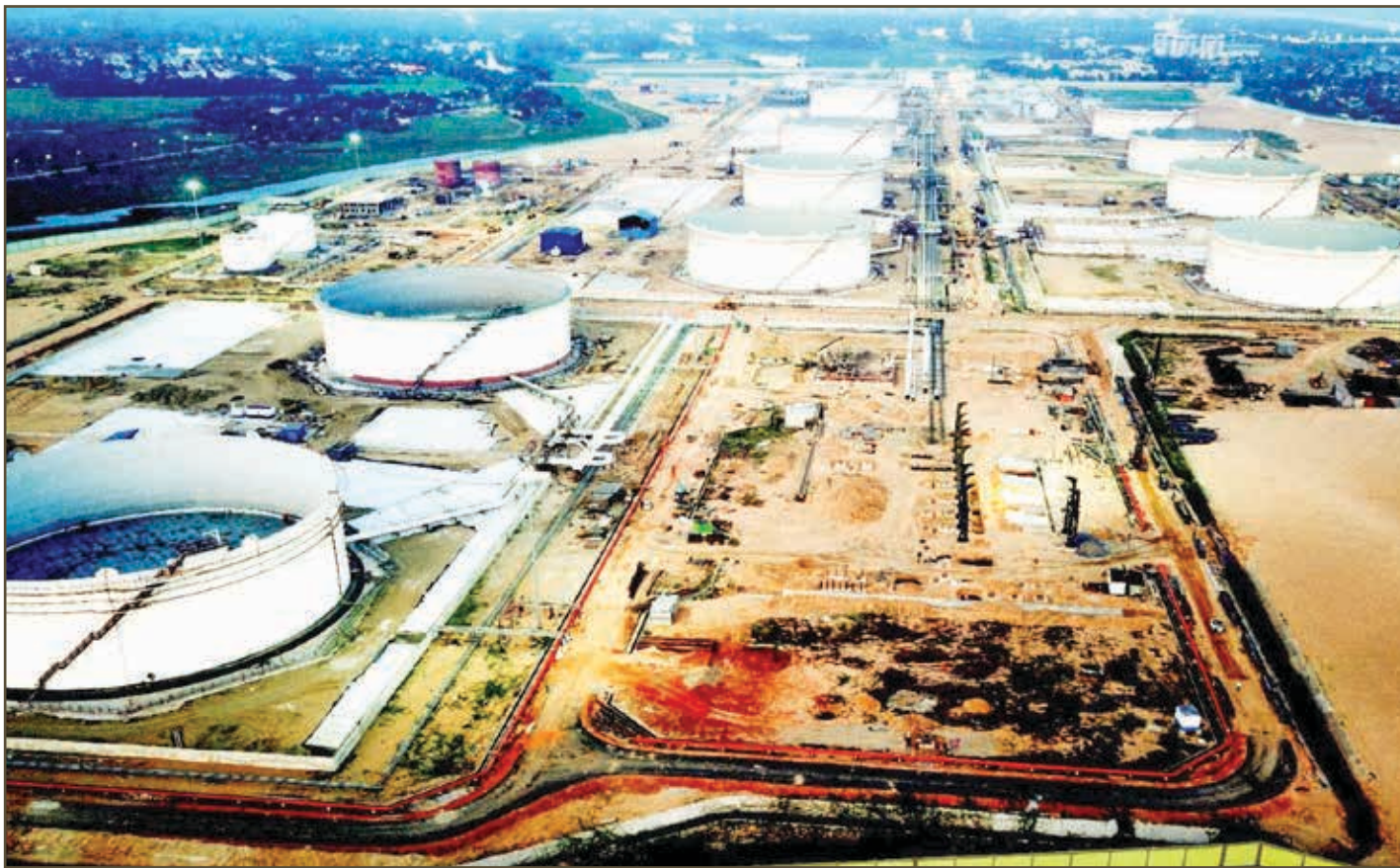
Bird's eye view of the Crude Oil Import Terminal (COIT) at Paradip Port
