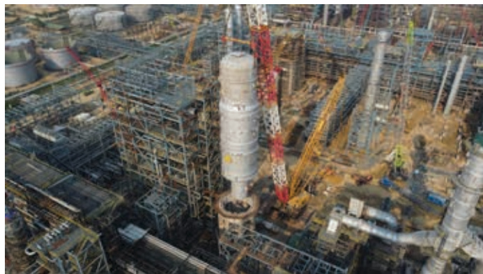
PFCC Main Fractionator Column Erection
