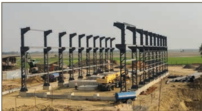
Erection of 20 columns of Mainline Pump House at IPPS-01, Bardhaman
