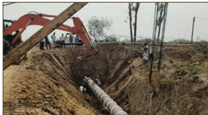
Cased Crossing Carrier Pipe Insertion under Kharagpur section of PNCPL
