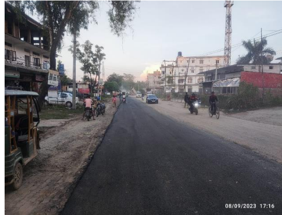
Telgaram Tiniali to Refinery main gate
