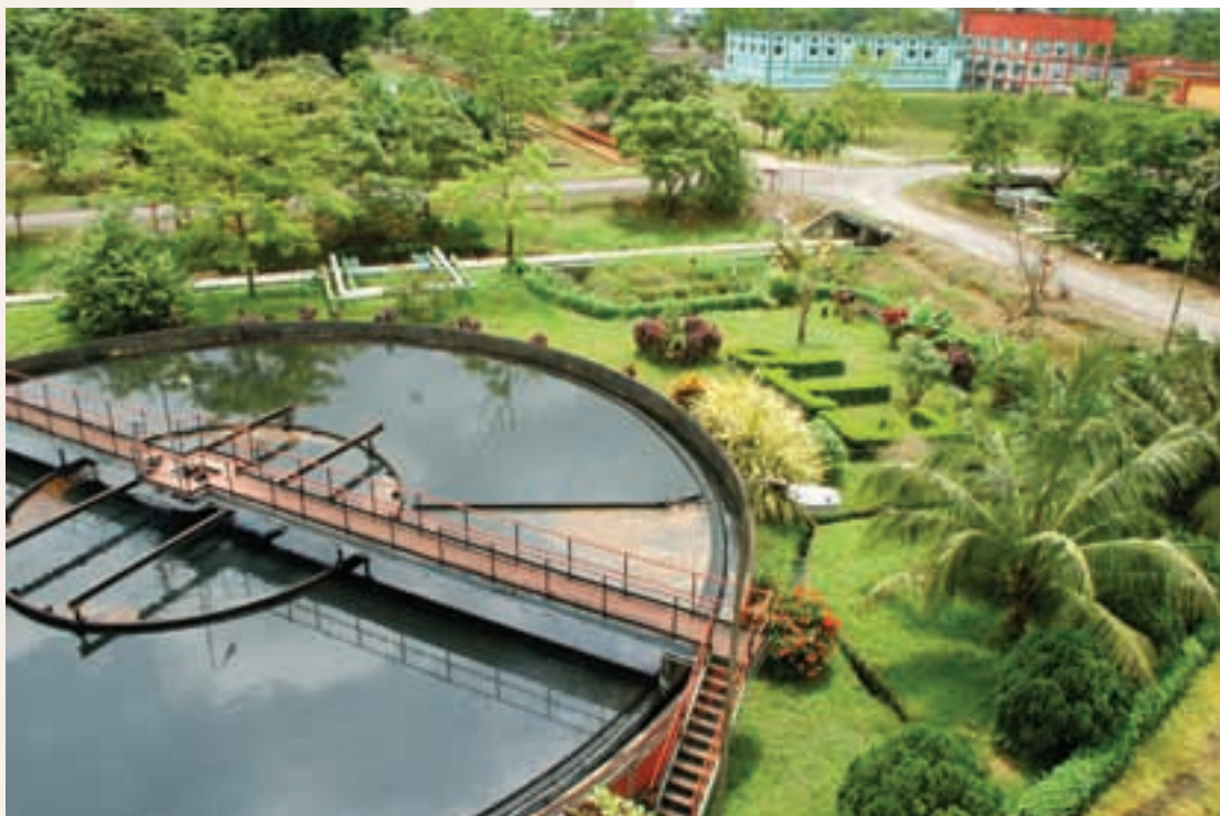
Effluent Treatment Plant
