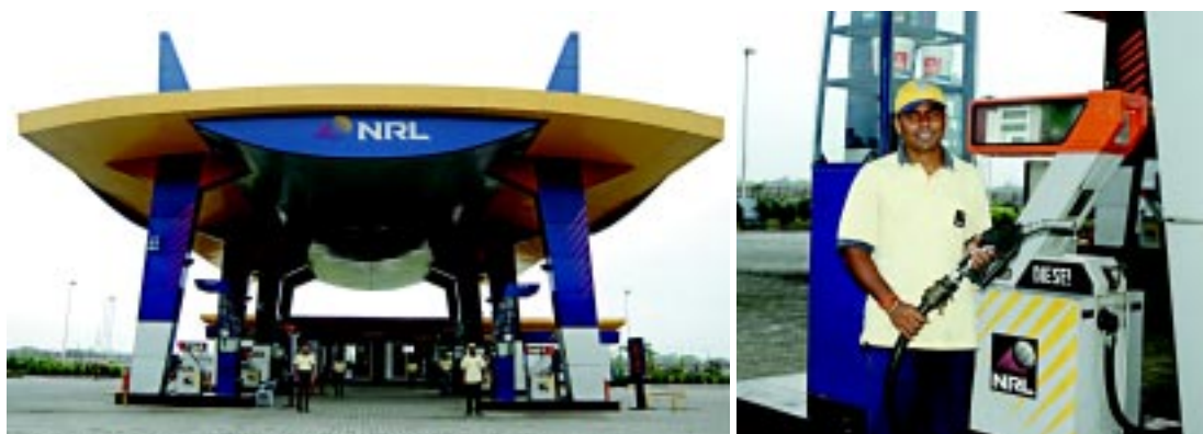
Energy Station of NRL
