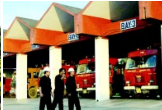
Fire brigade station
