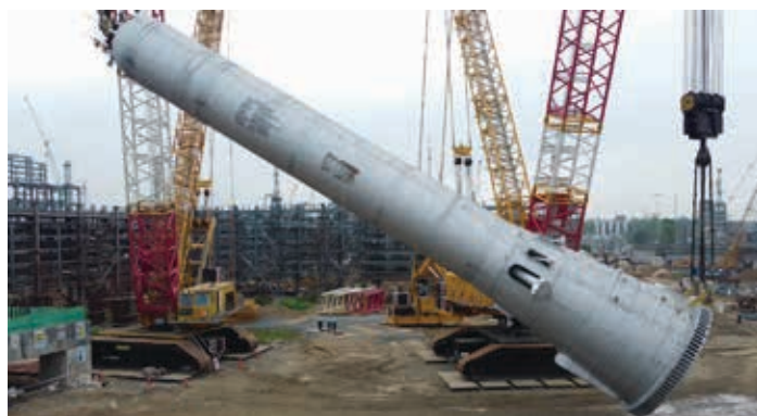
Transportation and erection of LC Finning Reactor
