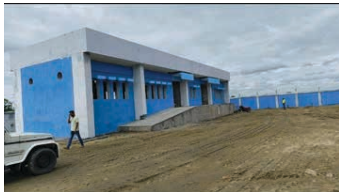
Painting work completed for Sectionalizing Valve Station (SV-61) in Assam. Slab Casting for other SVs viz: SV 54, 71, 75, 81, 83 and Repeater Station building completed in this quarter.
