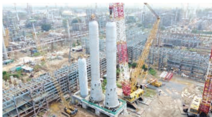
Transportation and erection of LC Finning Reactor
