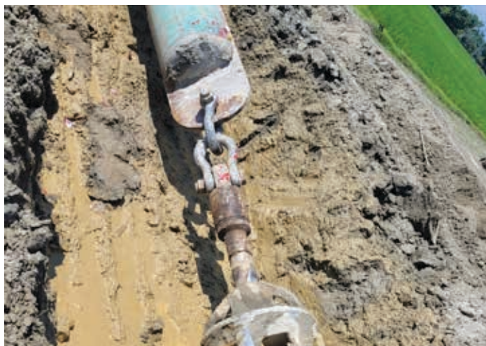
26 inch HDD pulling at Kaljani river
