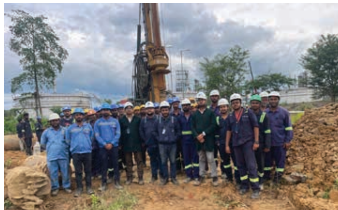
Piling job in Receipt Terminal (RT) in Numaligarh of PNCPL started on 2 nd August 2024
