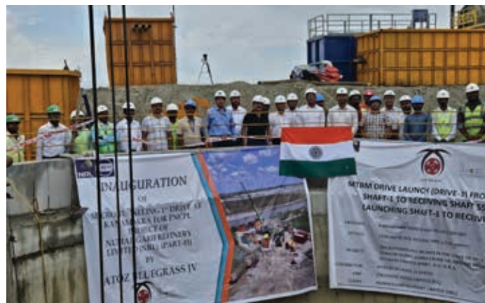
The 1 st Microtunneling drive started at River Guruphela for a section length of 500m in Gossaigaon, Assam section on 12 th August 2024
