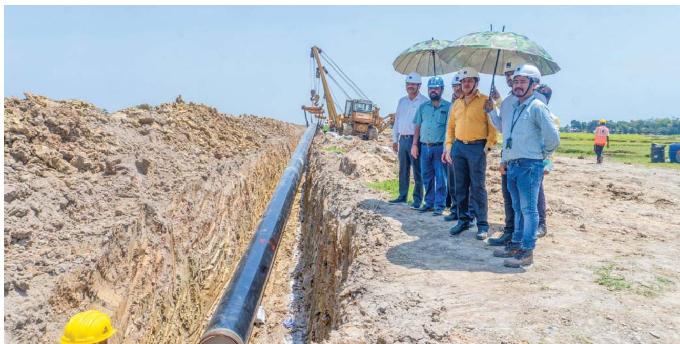
Laying of Crude Oil Pipeline for Numaligarh Refinery Expansion Project
