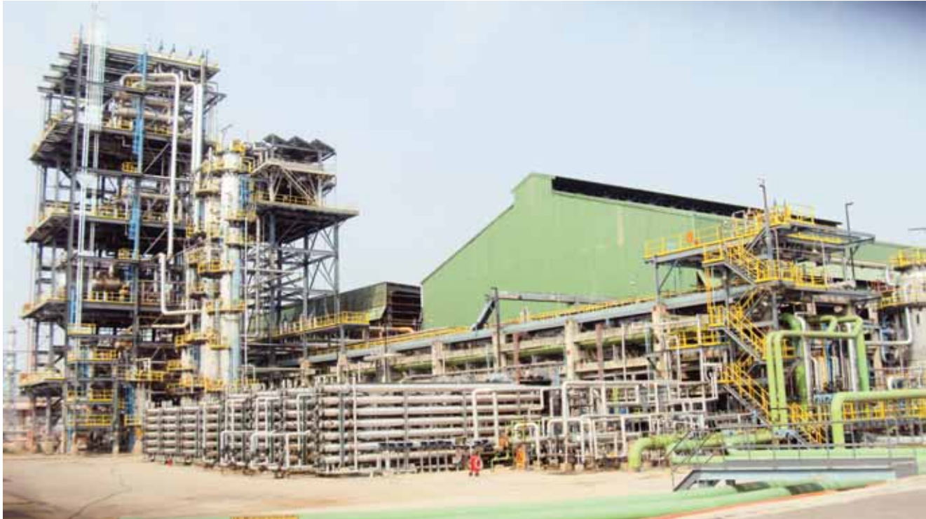
Solvent De-oiling Unit of WAX Plant
